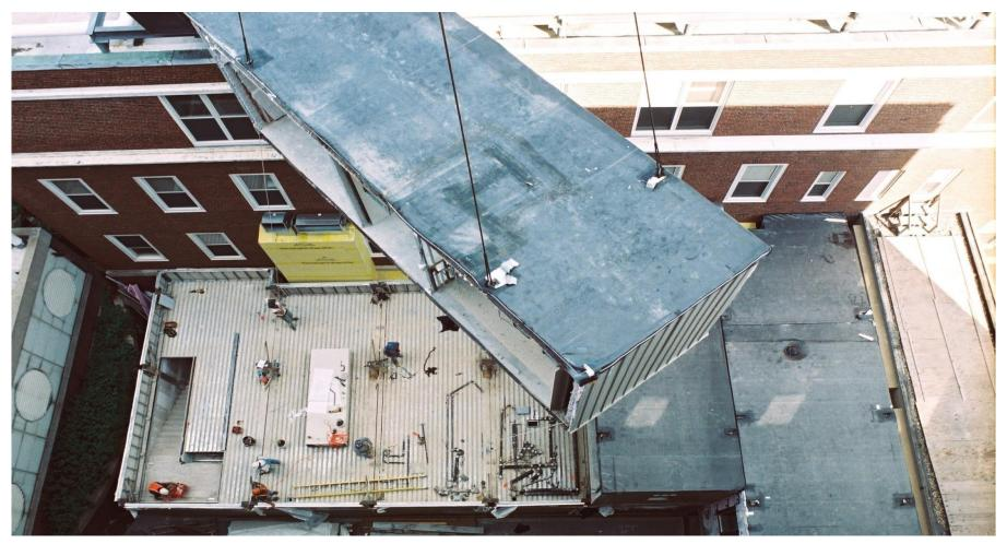
Steel and concrete modules are heavy and sizes can also be dictated by height and reach of delivery
