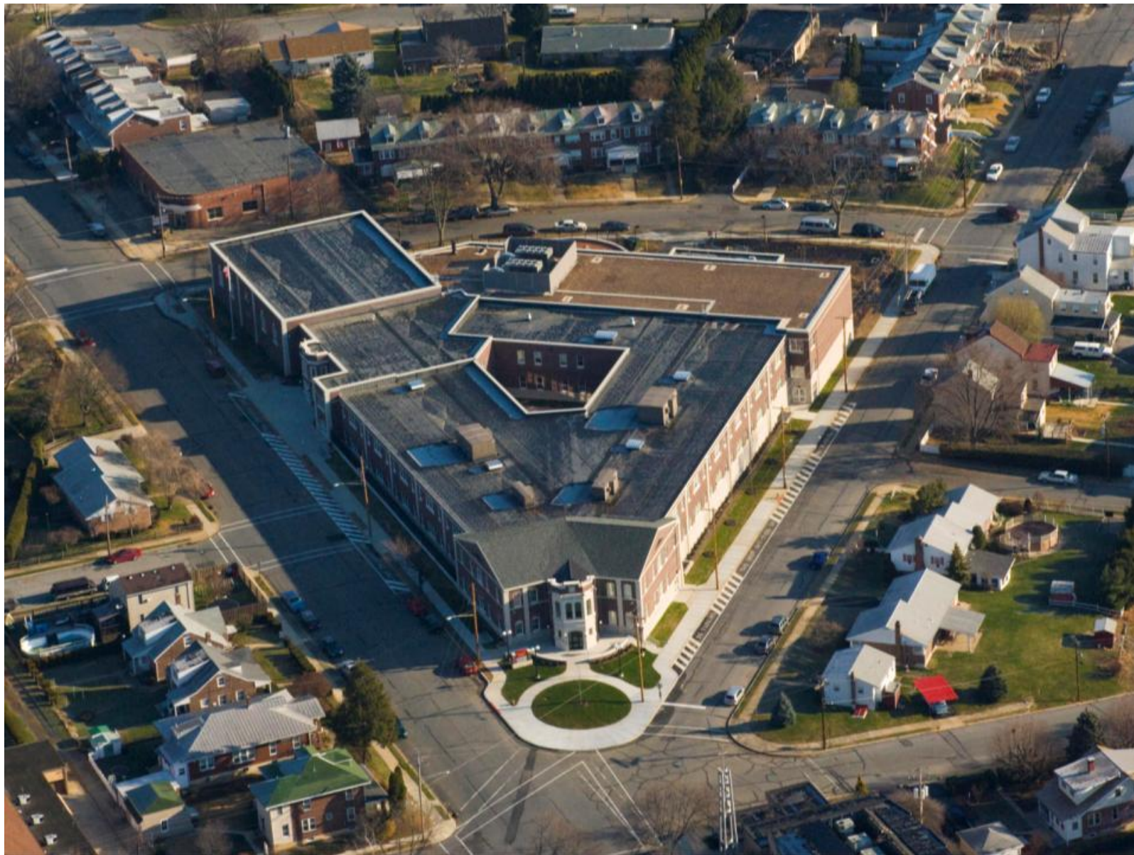
Reading School District – Millmont Elementary School RB
