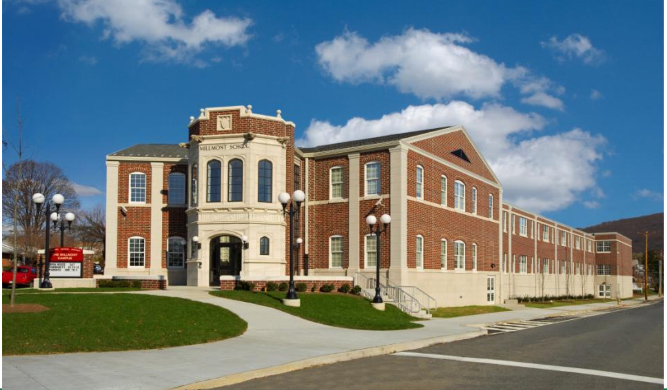
Reading School District – Millmont Elementary School RB
