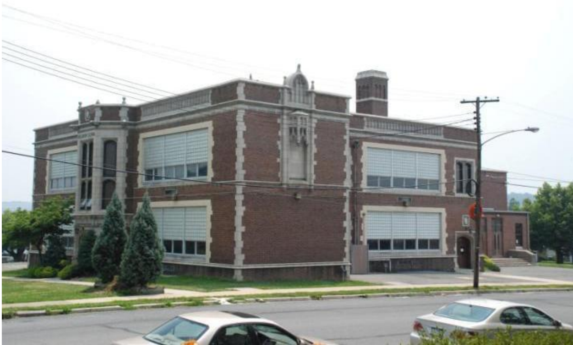
Reading School District – Millmont Elementary School RB
