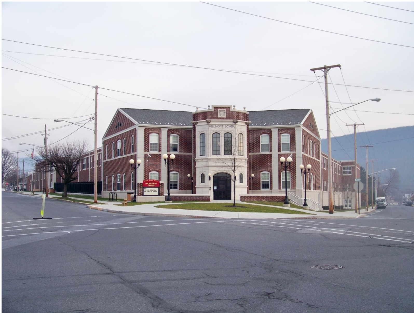
Reading School District – Millmont Elementary School RB
