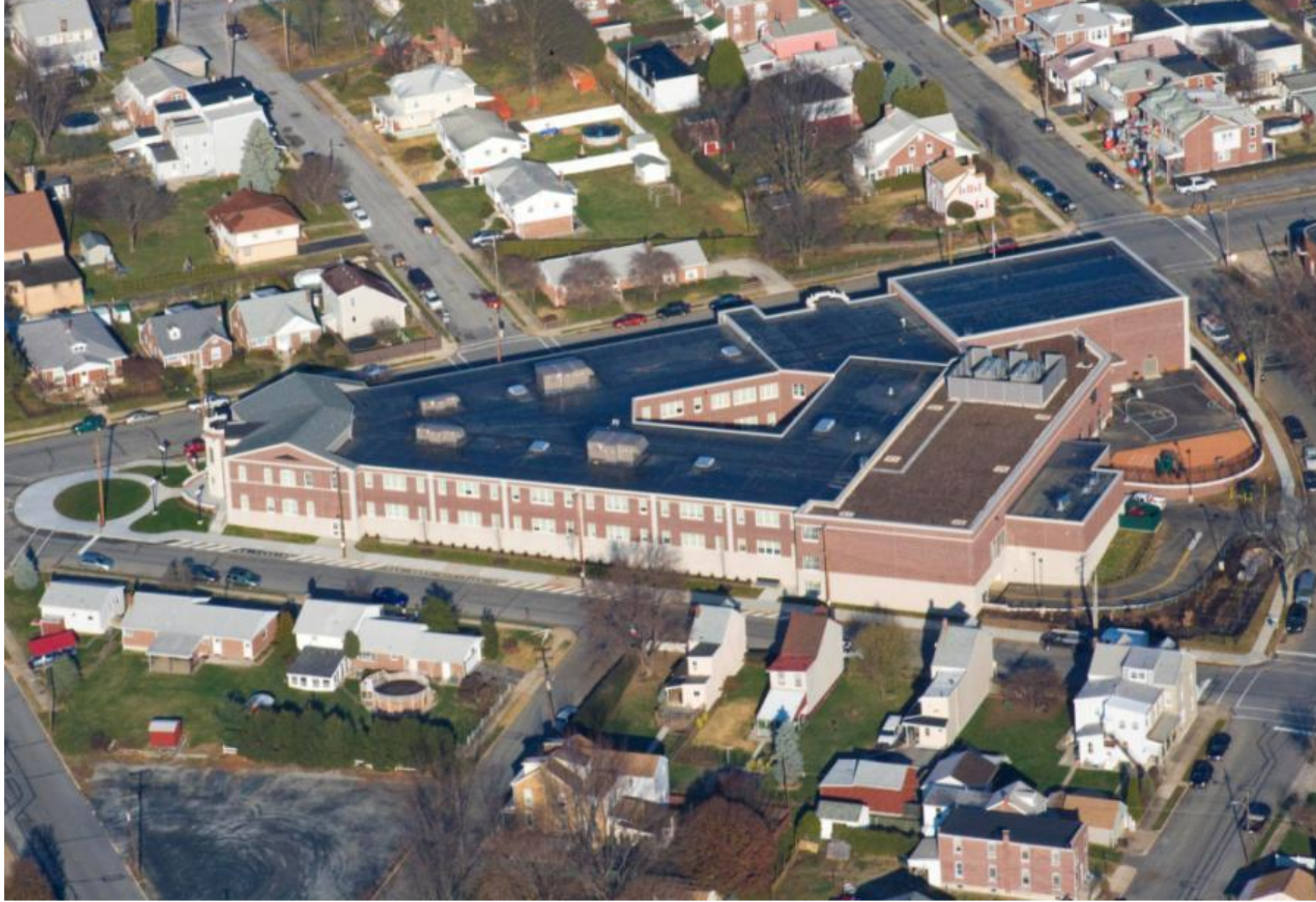
Reading School District – Millmont Elementary School RB
